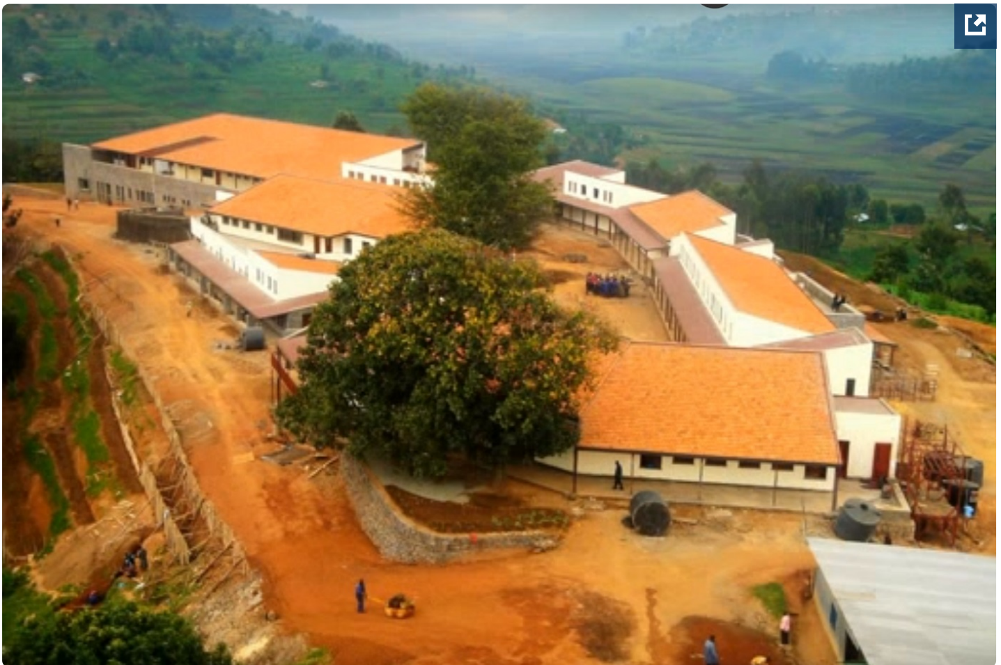
Butaro Hospital in Rwanda. In 2011, doctor's quarters were built here for US doctors to train and teach Rwandan doctors as well as provide care.
